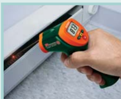
Test for temperature in heating systems
